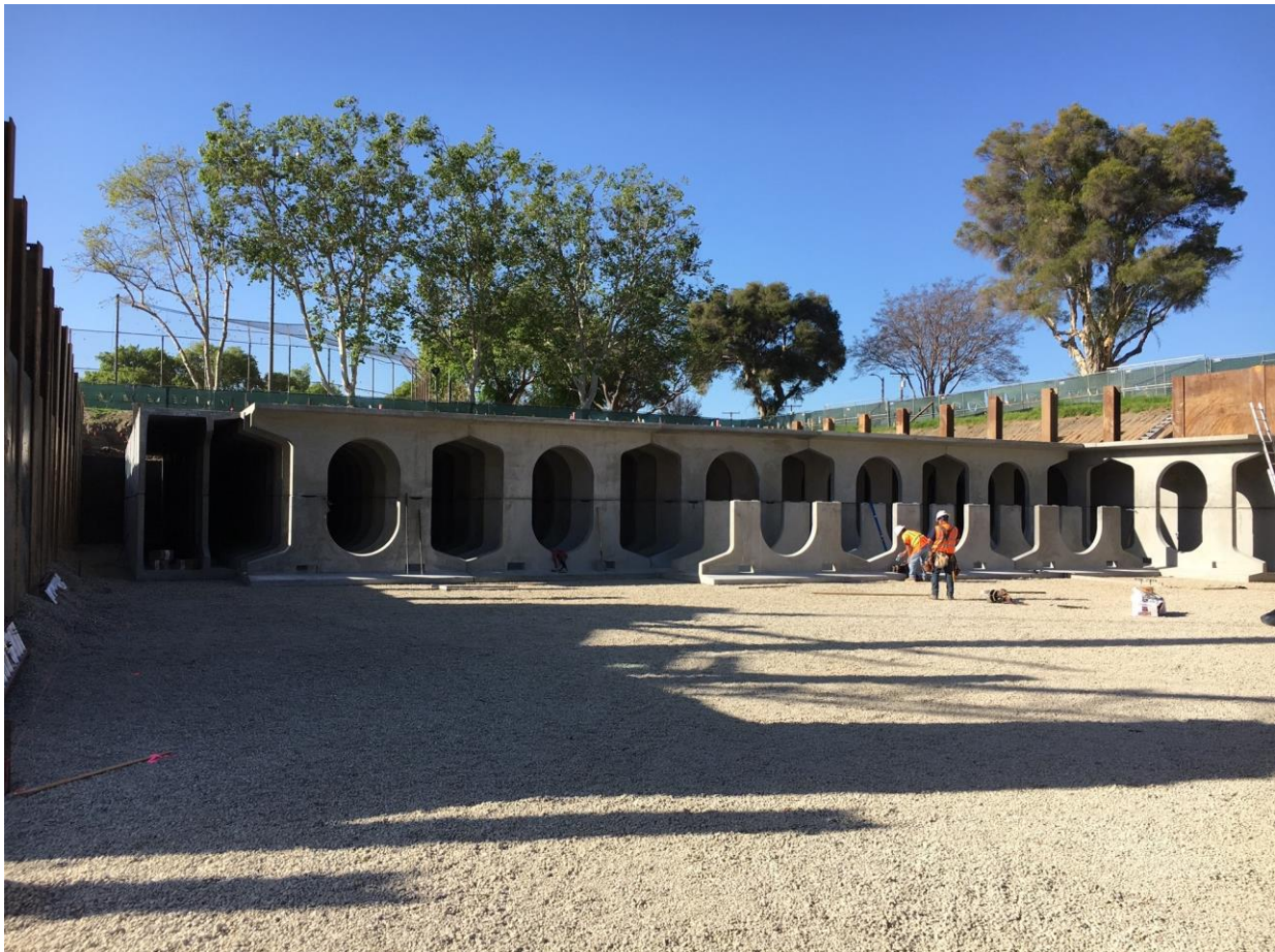
Figure 2-7. StormTrap Installation at Bolivar Park BMP
