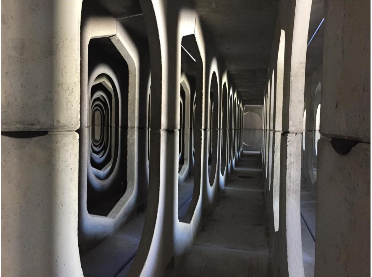
Figure 2-8. Inside StormTrap Unit Installed at Bolivar Park BMP
